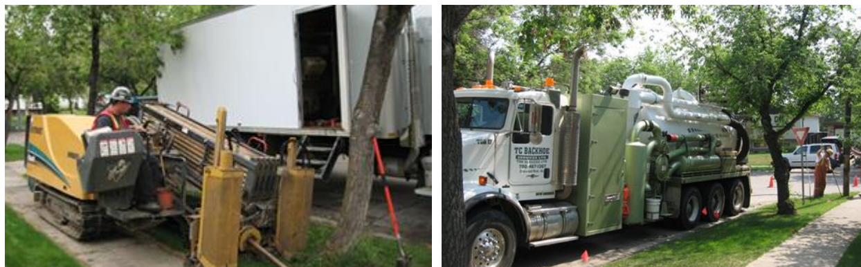
Figure 12 Directional Drilling (left) and Hydrovac Services (right)
