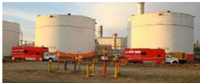
Figure 17 Storage Vessel Maintenance Opportunity
