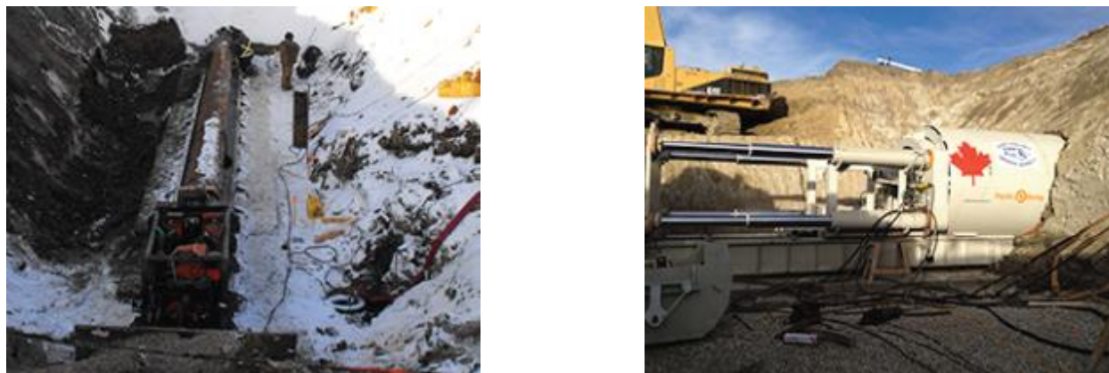
Figure 13 Horizontal Augering (left) and Pipe Jacking (right)
