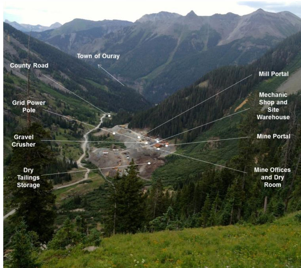
Revenue Mine – Surface Infrastructure
