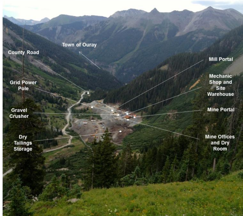
Revenue Mine – Surface Infrastructure
