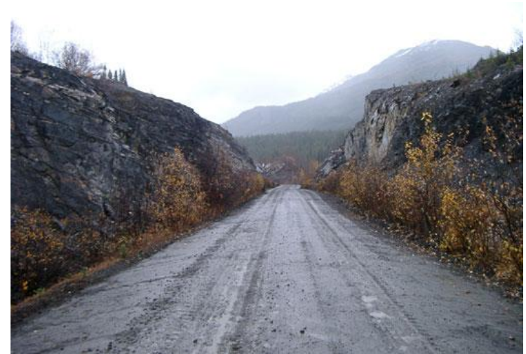
Existing railway right-of-way & road bed
