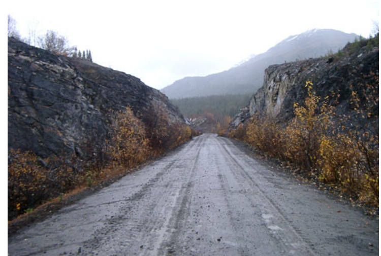
Existing railway right-of-way & road bed
