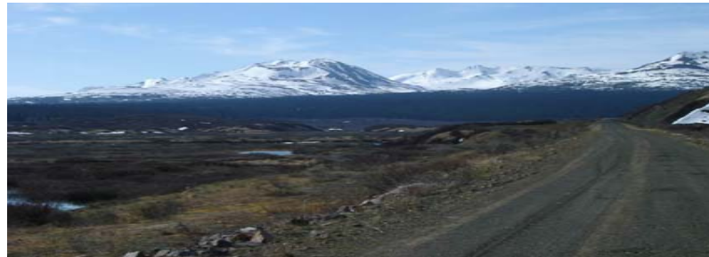
Railway sub-grade links mine site with CN mainline & Ridley Terminals
