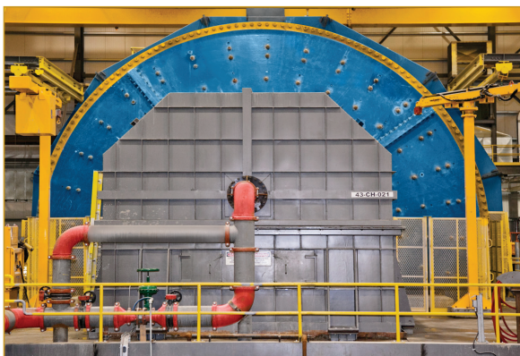
New Mill expansion at the Endako Mine, British Columbia
