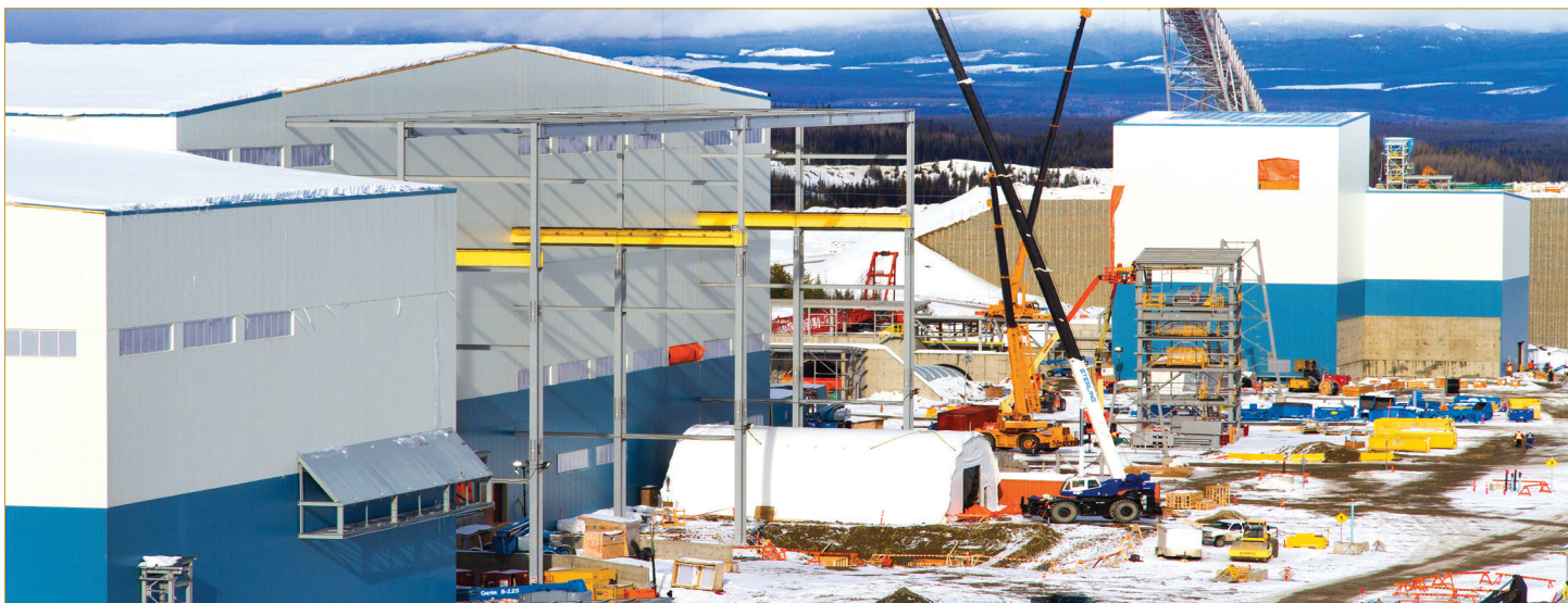
Truck shop, warehouse and administrative buildings at Mt. Milligan, British Columbia
