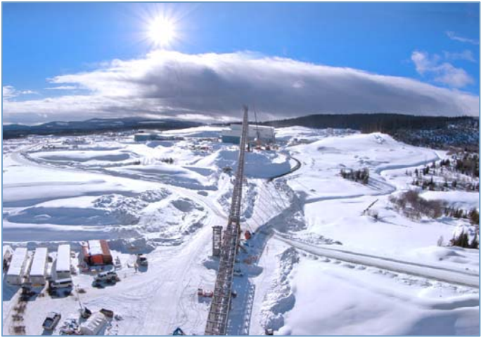
Conveyor from primary crusher to course ore stockpile
