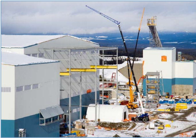
Concentrator building and pebble crusher
