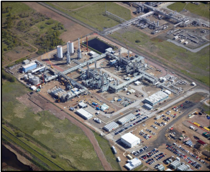
Teesside Gas Processing Plant
