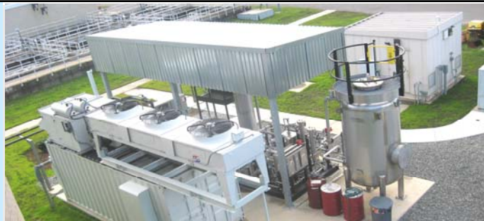
Biogas System at the Village of Ridgewood Water Pollution Control Facility
