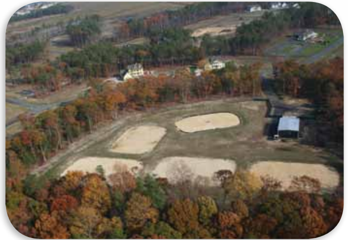
Wastewater is treated to a high level effluent quality and disposed of through rapid infiltration basins which help recharge the aquifer.
