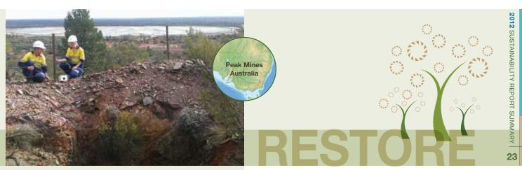
Inspection of one of the historic mine shafts within Peak's mining leases. In 2012, 49 shafts were inspected for safety and environmental risks and bat habitat. We also evaluated fencing, signage and fill requirements.
