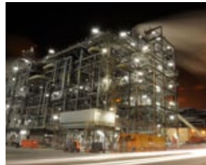
QATAR: PEARL GAS-TO-LIQUIDS PLANT
