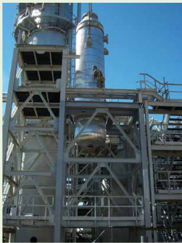
Depropanizer reboiler being set
