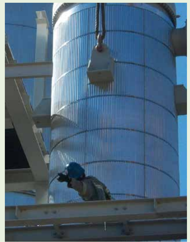
Final work on depropanizer reboiler
