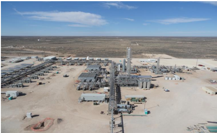
200 MMCFD Driver Plant (WestTX) – April 2013
