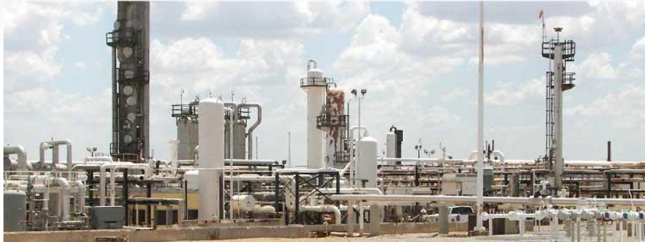
60 MMCFD V-60 Plant (SouthOK) – April 2012
