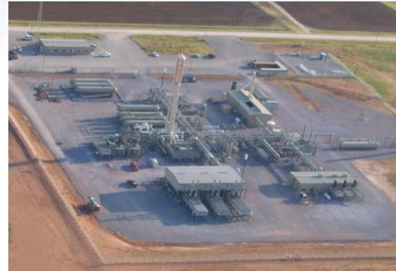
200 MMCFD Waynoka II Plant (WestOK) – September 2012
