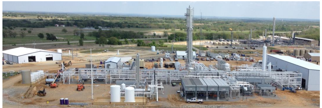
120 MMCFD Stonewall Plant (SouthOK) – May 2014
