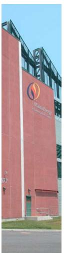
The Marina Thermal Facility (MTF) is our largest project, providing the Borgata Hotel Casino & Spa (along with its Water Club expansion) with electricity, heated water, and chilled water used for lighting, power, air conditioning, space heating, and domestic hot water production. MTF can also provide electricity to the casino and the PJM grid during periods of emergency and peak electricity demand.
