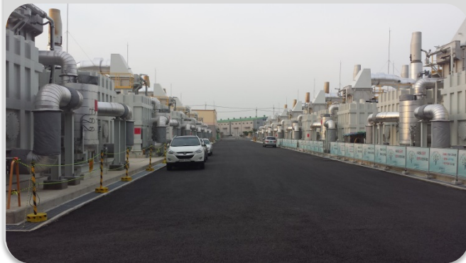
59 MW fuel cell park under construction
