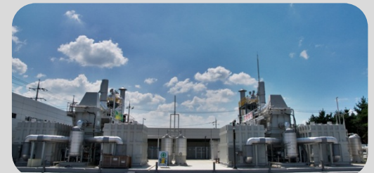
Fuel cell park supporting the electric grid
