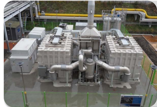
2.8 MW power plant
