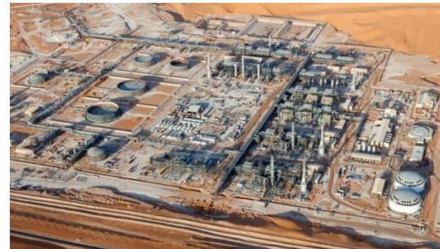
El Merk gas processing facility, Algeria
