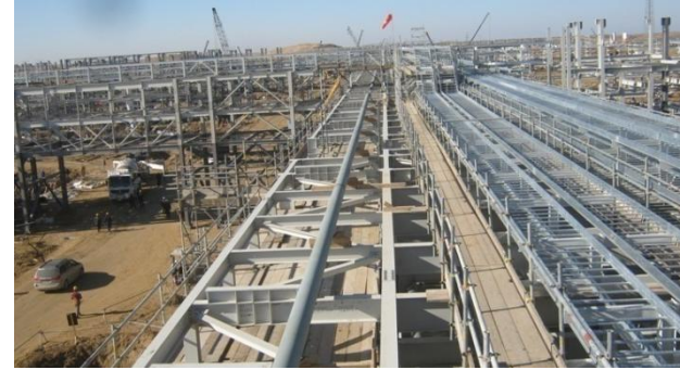
South Yoloten gas field development, Turkmenistan
