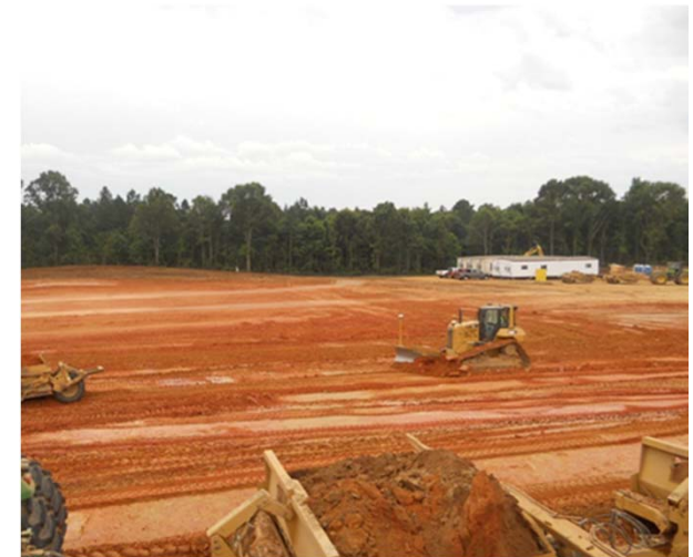
Amite Site – Ground Clearing (July 2013)
