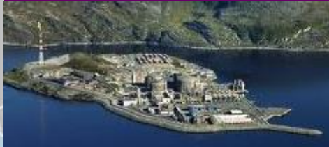
Land based 2 train LNG plant
