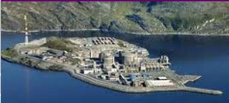
Land based 2 train LNG plant
