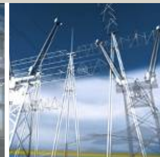
High-voltage switch gear
