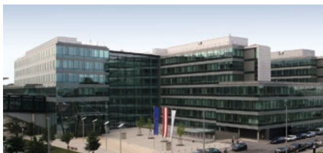
Office Campus Gasometer | Vienna | AT
