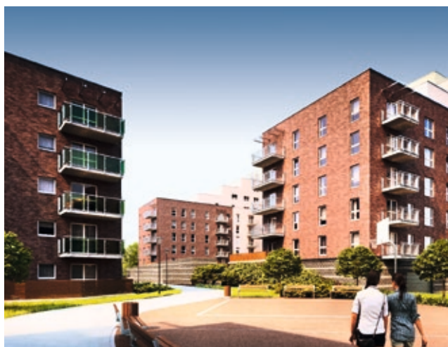
Dębowe Tarasy Residential Estate | Katowice | PL
