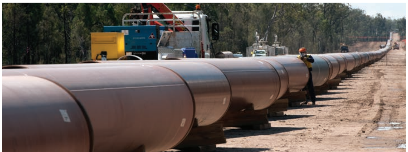
Main pipeline network for QCLNG project, Queensland, Australia
