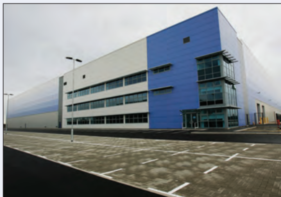
Unit 1, G. Park, Portal Way, Liverpool
