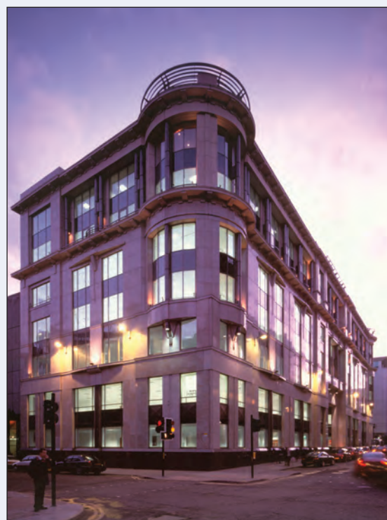
Alhambra House, Wellington Street, Glasgow
